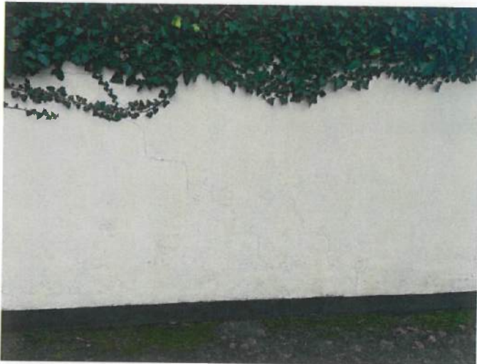
Fig 4.1 Structural cracks in End Wall Location 3
