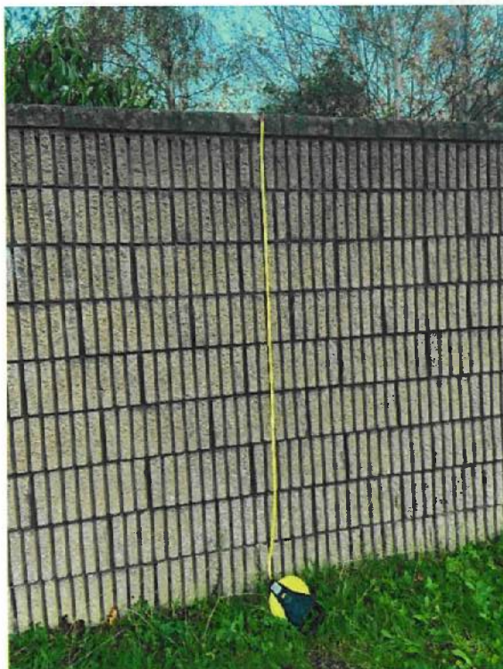
Fig 2.1 2m High Architectural Masonry Boundary Wall (View from R132)
