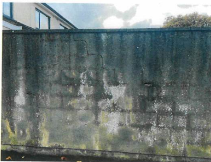
Fig 4.1 Structural cracks in End Wall Location 3
